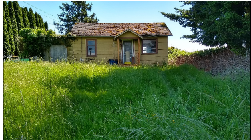
Photo 8. Existing building on parcel P37251 from sample plot P12, facing south.
